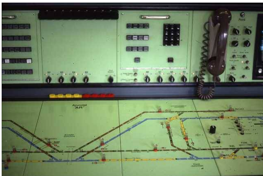
Figure 151 - Westinghouse M5 NX(PP)[+], Arundel. © CJ Woolstenholmes
