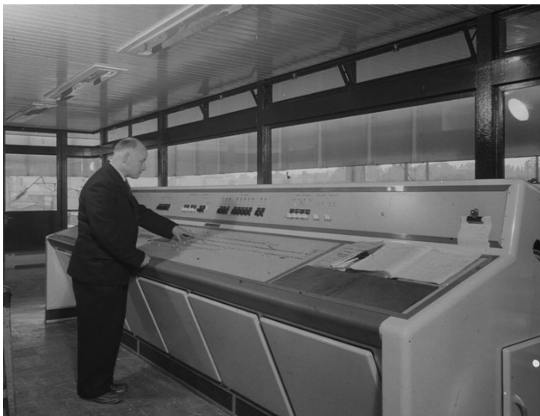
Figure 136 - Westinghouse NX(PP)[+], Broxbourne. © Siemens.
