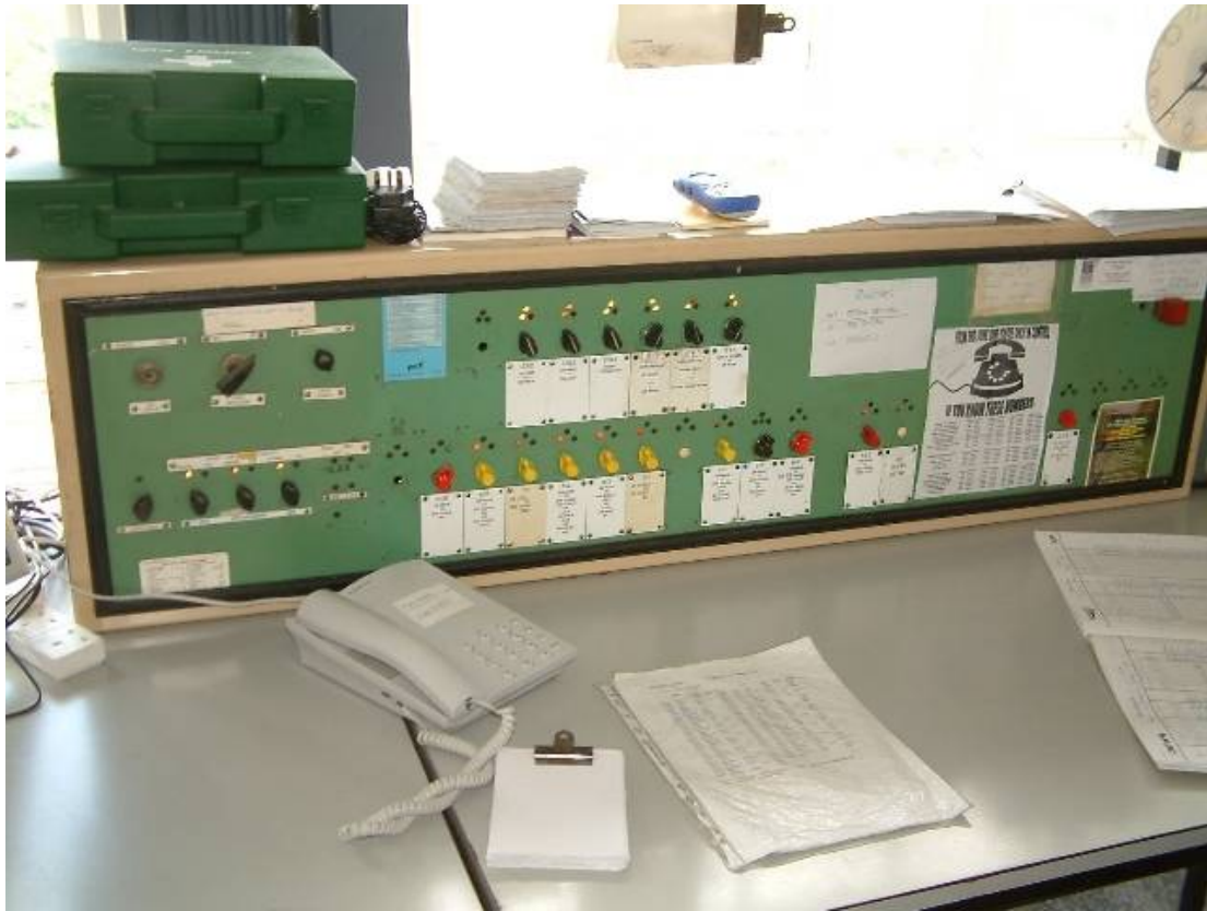
Figure 147 - Westinghouse M2 IFS[-], Bowesfield (Eaglescliffe Panel). © John Midcalf
