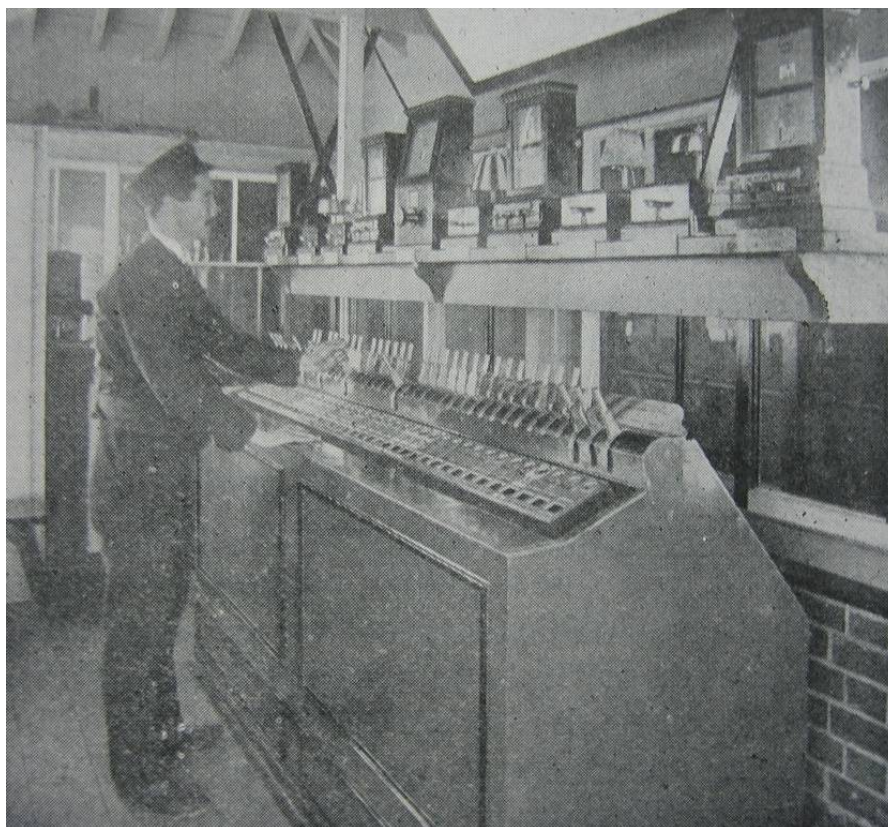
Figure 171 - Siemens All-Electric PF(L), Didcot North.
