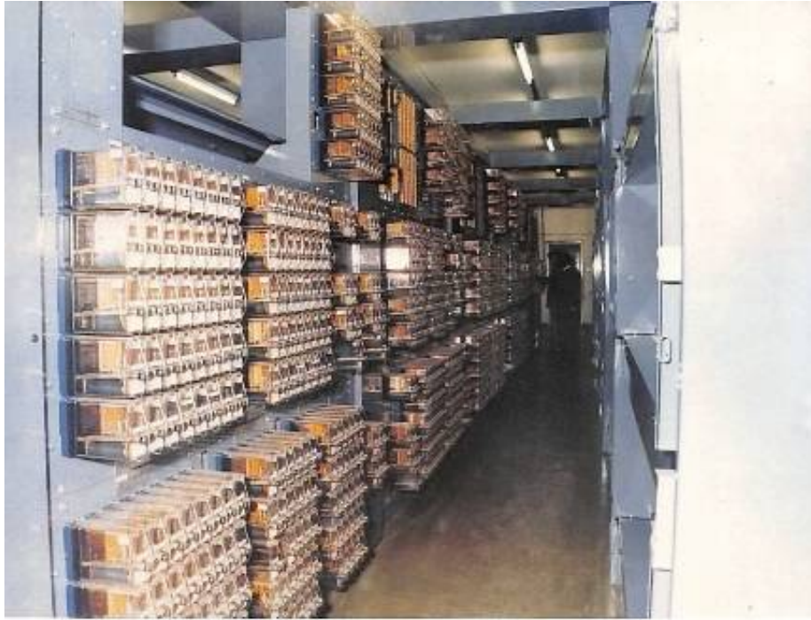
Figure 198 - Westinghouse Westpac MkIVA geographical interlocking, Bedford. © Siemens.
