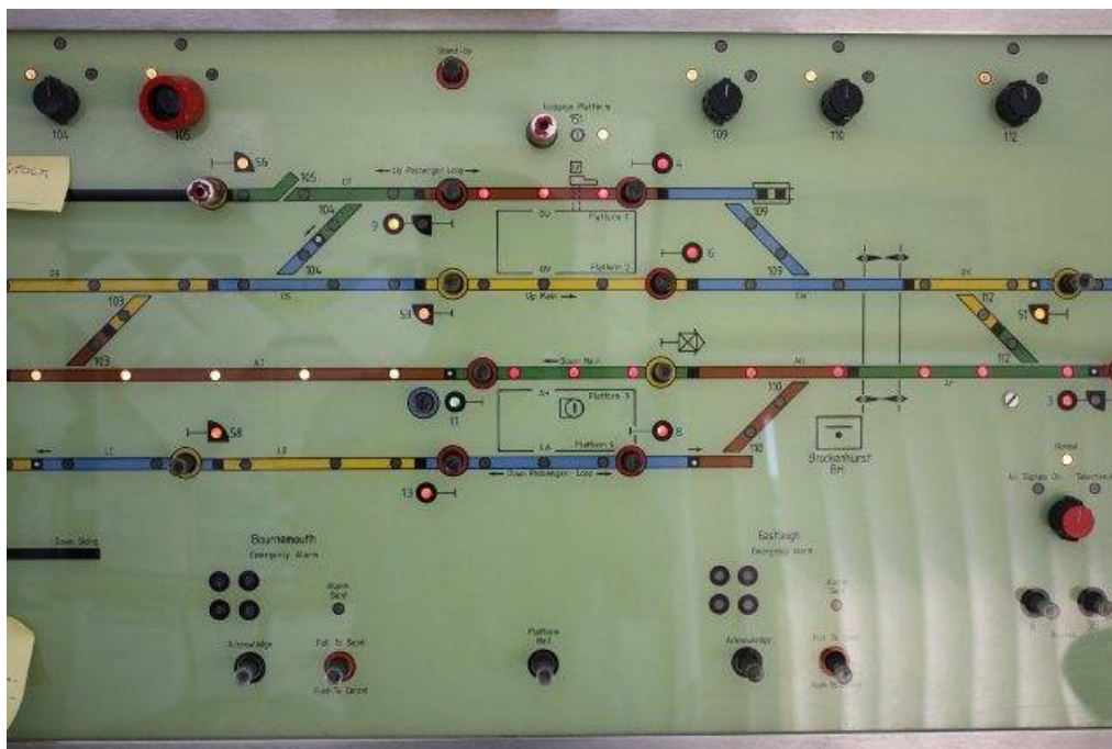
Figure 87 - ML Engineering NX(PP)[+], Brockenhurst. © Danny Scroggins
