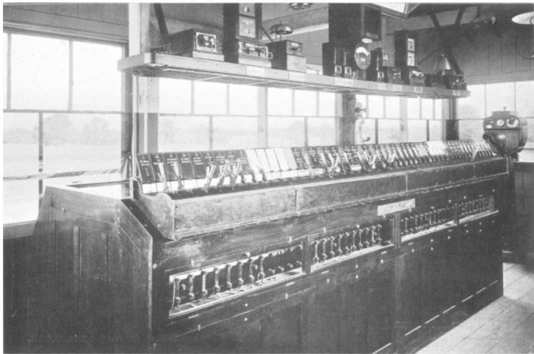
Figure 181 - Westinghouse M1 PF(L), Yarnton Jcn. © Siemens.
