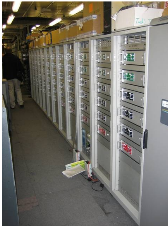
Figure 186 - Westinghouse (BRR) MkIIB SSI, Slough New. © Andrew K Overton.
