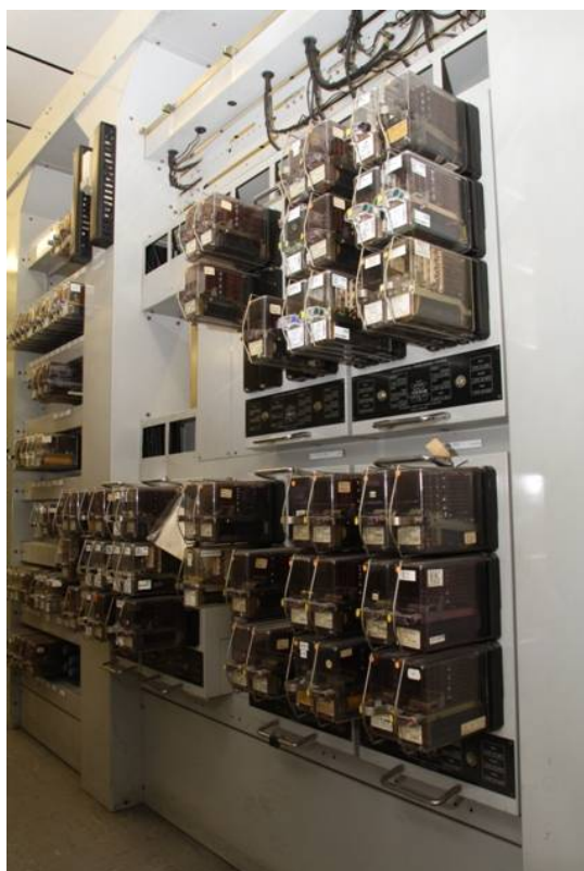
Figure 187 - GEC-GS geographical interlocking, Stewarts Lane. © Simon Foster.
