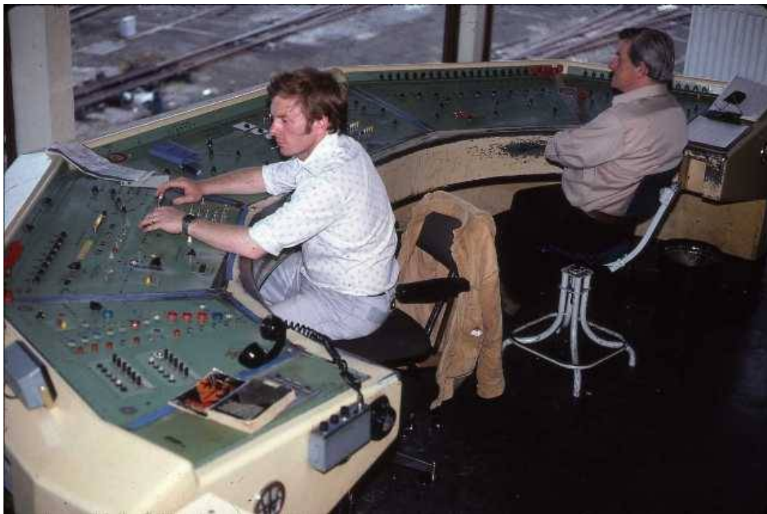
Figure 143 - Westinghouse MCD NX(PP) / IFS(Y3)[+] Hybrid, Tees Down Yard Control Tower. © CJ Woolstenholmes
