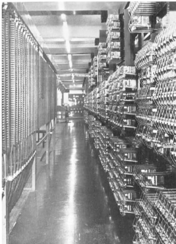
Figure 196 - Westinghouse Westpac MkIIIA geographical interlocking, Warrington. © Siemens.
