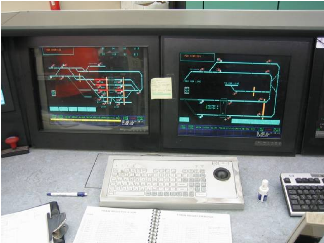
Figure 3 - ABB DCS WS, Drax PS FGD Control Room (Coal, Ash & Dust WS). © Andrew K Overton
